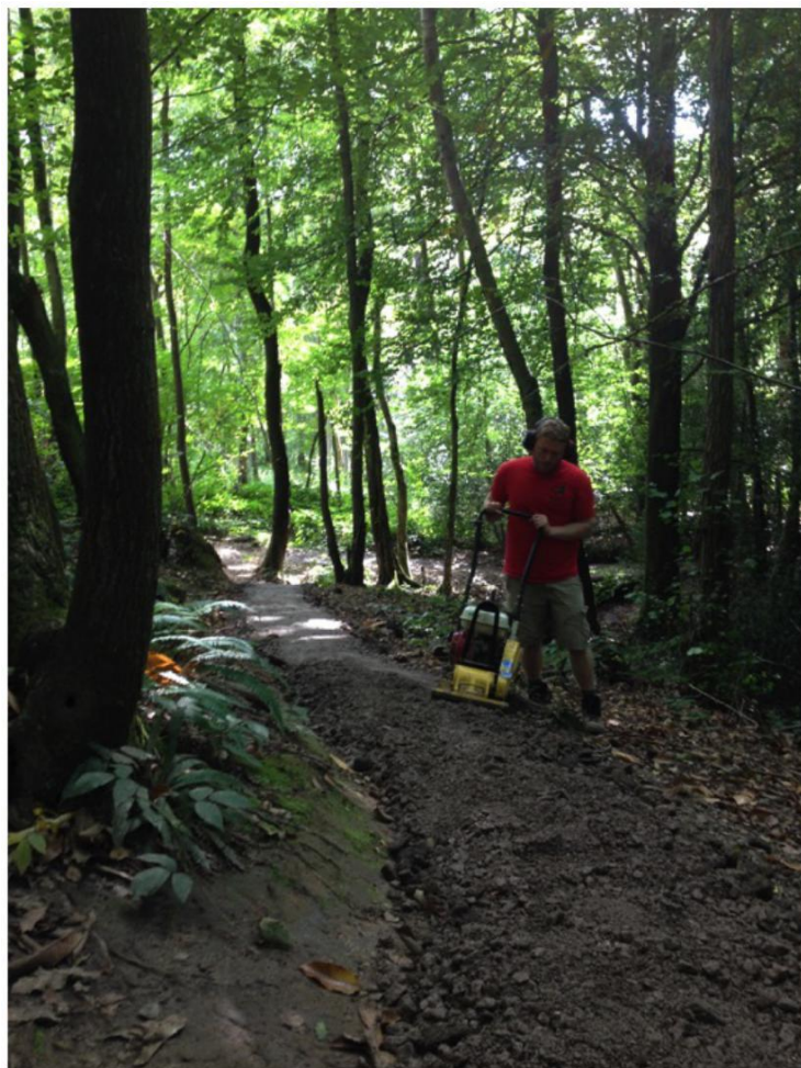
Phil using the whacker plate on the cycle trail
